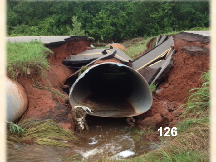
Undermined 6" Dowel Jointed PCC Pavement. Photos show loss of subgrade, separator fabric and buckling of surface
